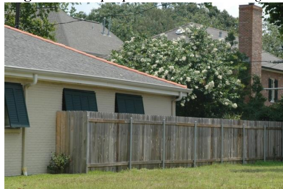
Figure 12 Improper – external bracing
