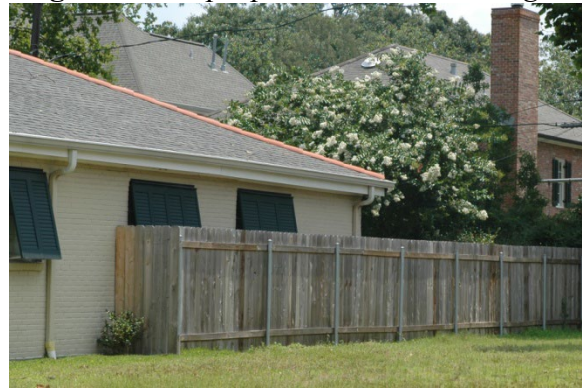
Figure 12 Improper – external bracing
